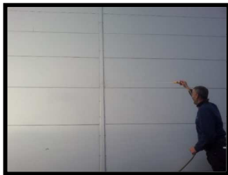
Water testing of the architectural wall panels
